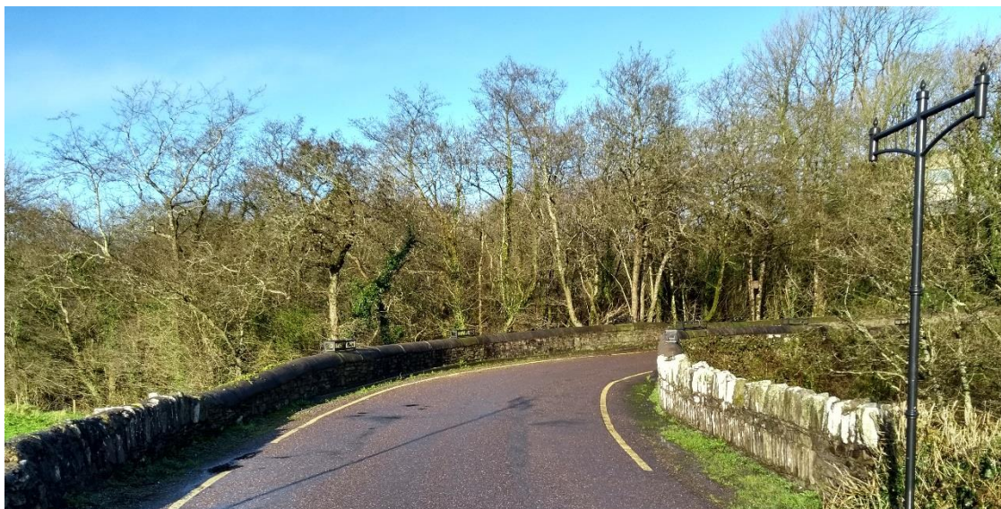
Figure 8 The stone bridge at Ballinora.
