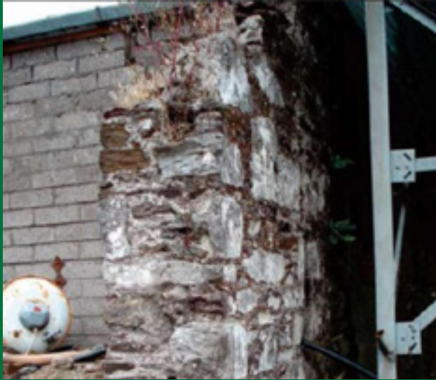
Part of the wall of the original farmhouse
